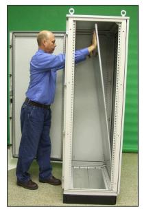
D) Continue to push the top of the panel until the collar studs protude through the panel mounting holes. Ensure the pins protrude through the bottom of the panel supprts.
