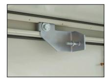
B) Secure the bottom panel supports and the upper panel mounting brackets into place. To make sure the inner panel is straight, line up the back face of the upper mounts to the back face of the bottom supports.
